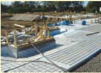
Left, concrete/eps slab-edge insulated forms and sub-slab insulation on FPSF for an elementary school in Stockholm, Sweden. In Norway, Sweden and Finland, 2-inch thick sub-slab insulation, either EPS or XPS, is widely used under concrete slabs to keep the concrete warm for thermal comfort. BPA Construction.
