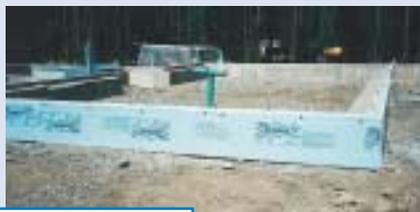
But with a FPSF, the footings only have to be 16 inches deep. With FPSFs as an option, the full basement is an expensive premium: \$10,000 to \$15,000 more than the same house built on a slab with an FPSF."
