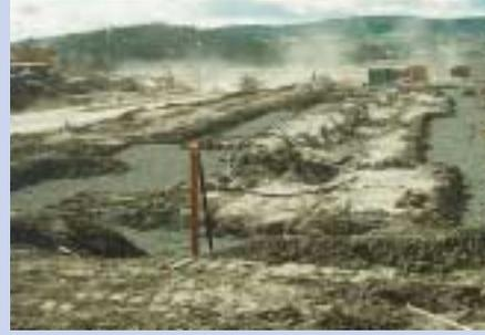
**Right:** Townhouse excavations showing gravel in trenches and utility preinstallation, prior to forming of grade beams, Oslo, Norway (Moelven Construction)
